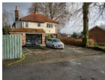
Cornerstone House, Sandbach
